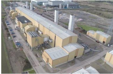
2 Battery 50 MW in Brigg, UK
