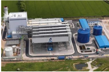
3 CCGT 445MW Whitegate plant in Cork, Ireland
