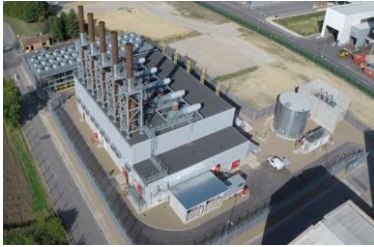
2 Gas peaking plant 50 MW in Brigg, UK
